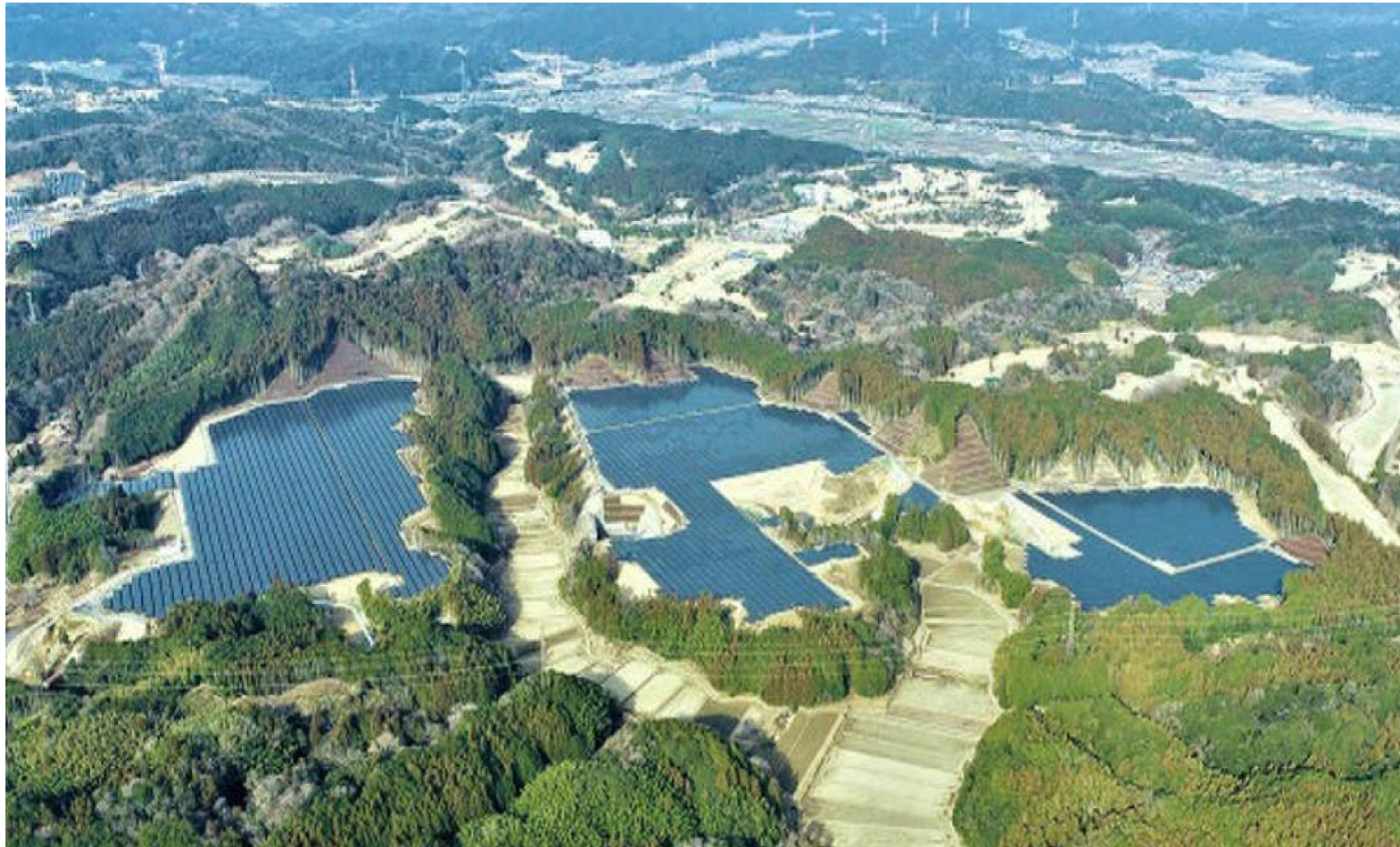
Power Plant Tsunamase 50MW
