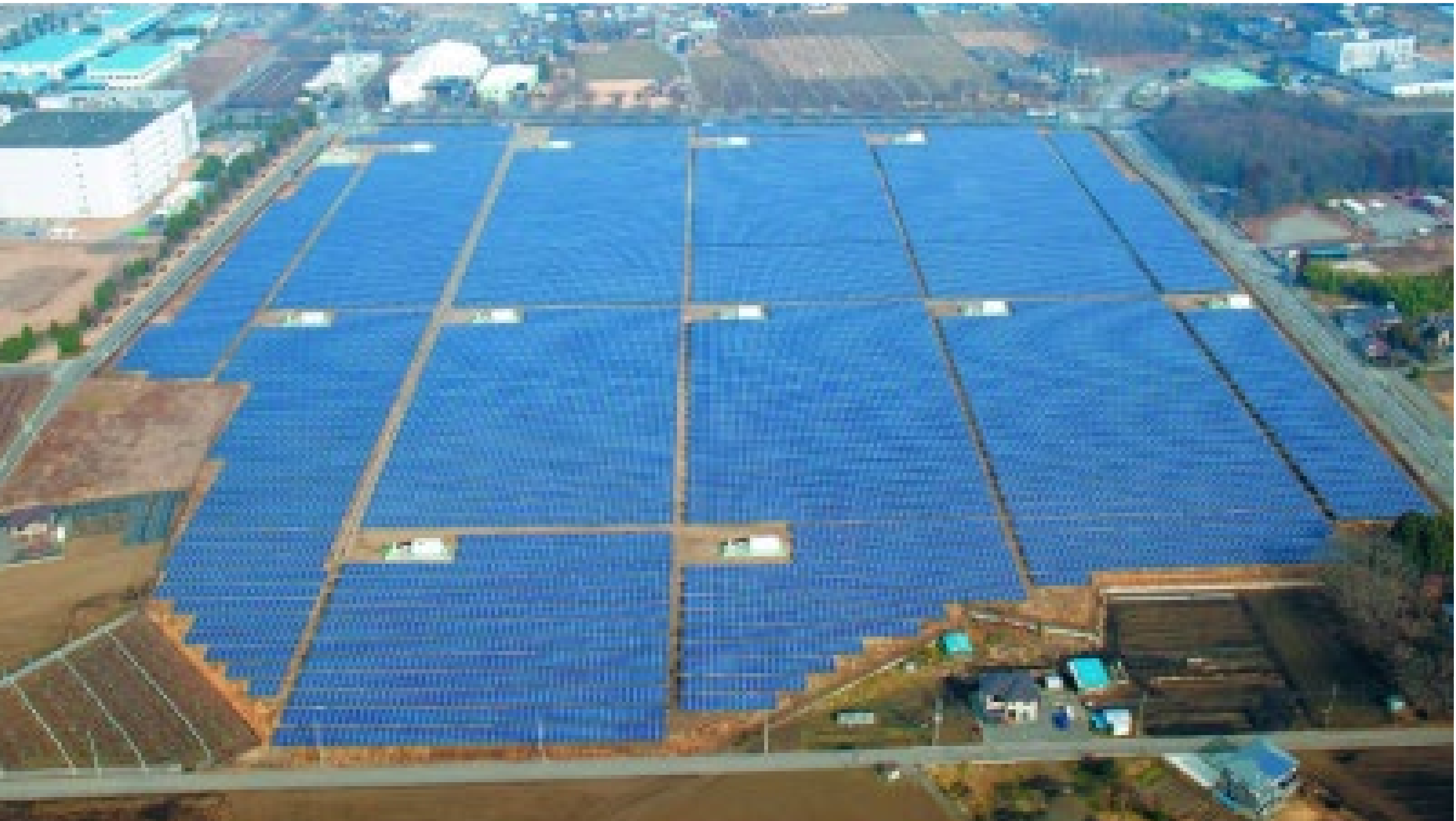
Tochigi Power Station 13MW
