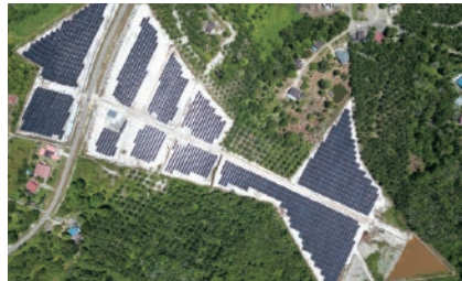
System capacity: 7MW Beaufort, Sabah Malaysia
