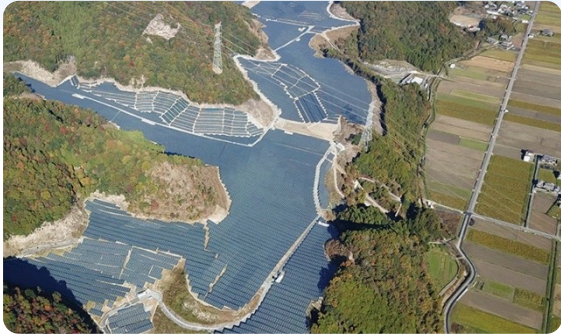
72.4MW, Japan Himeji Hyōgo Solar cable
