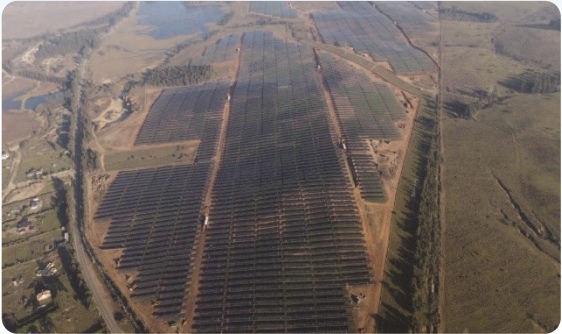
95.2MW, Chile Valparaíso Region Solar cable
