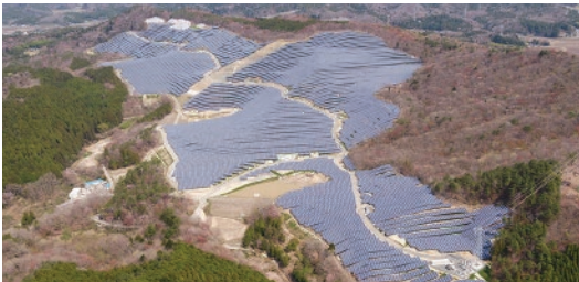
System capacity: 42.3MW Japan
