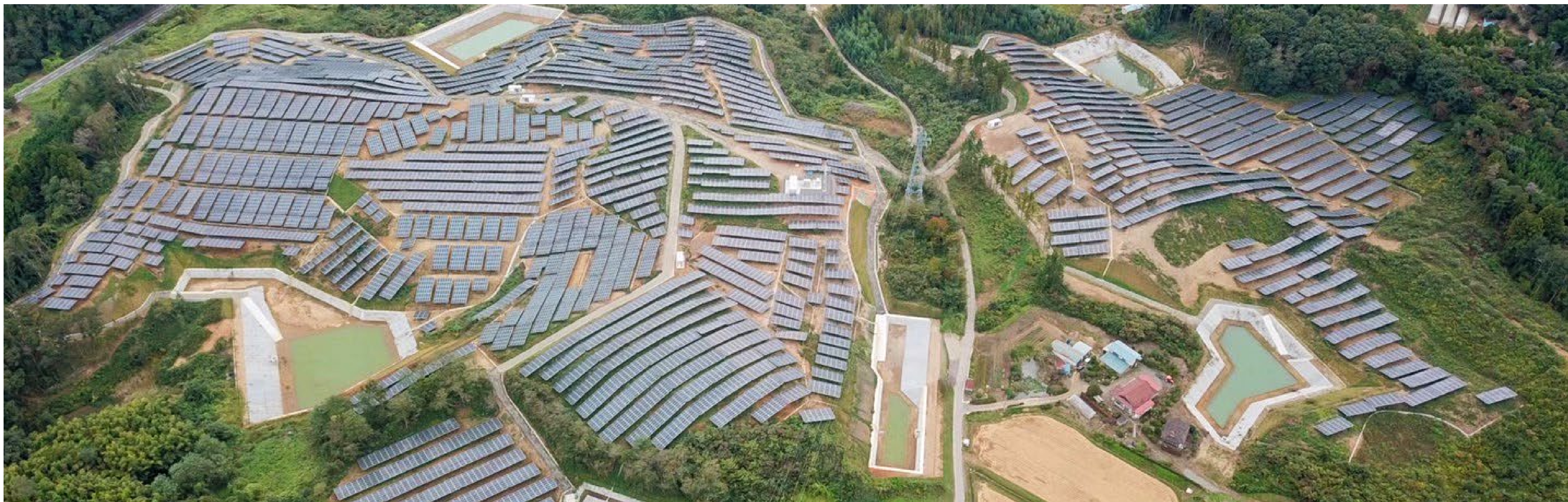
Suimei Solar Park 52MW
