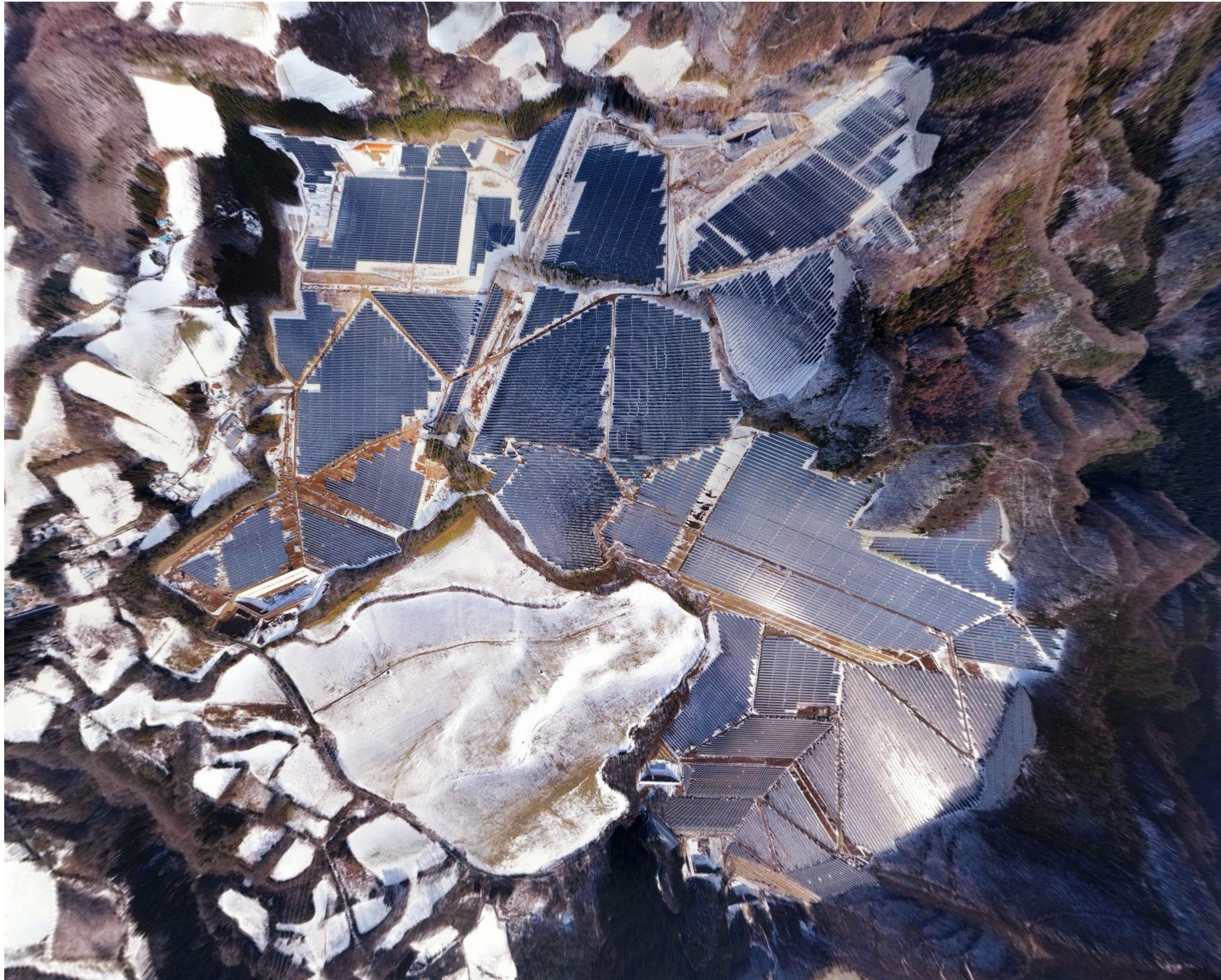
Shiraishi Solar Farm 162MW
