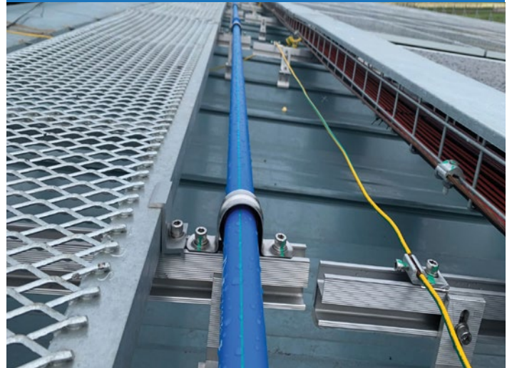
Cleaning Water Supply System
